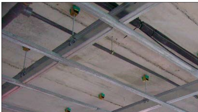
Application of an Akustik 4+Sylomer 30 type A
