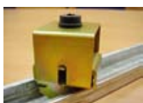
1. Place the part inside the beam.
