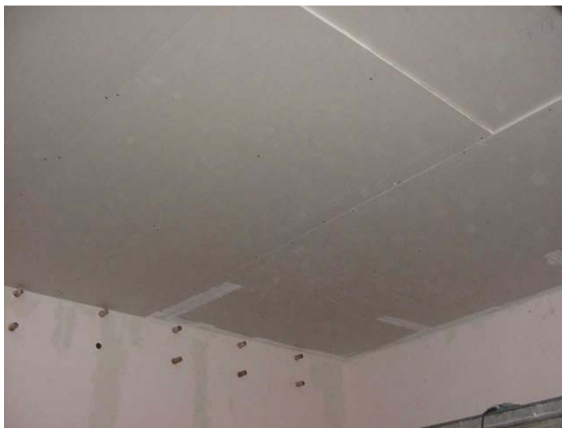
Photo 4: Mounting of the third plasterboard
