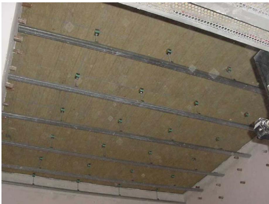
Photo 3: Mounting of the ceiling supports and the metallic profile
