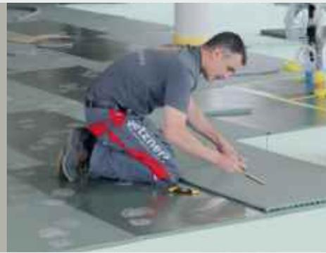
Using the Getzner Acoustic Floor Mat enables a rate of impact noise reduction of 33 dB
